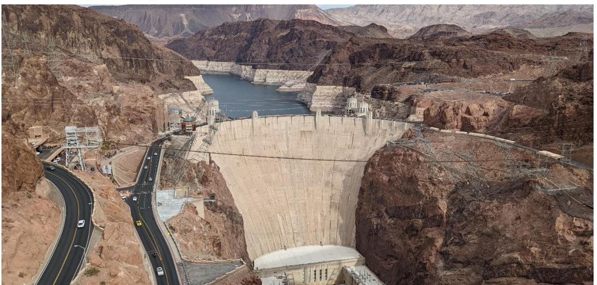
15 Hoover-Dam, Nevada November 22
